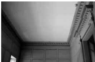
Drayton Hall stair passage ceiling.
